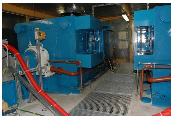
Figure 2: Two fly-wheel generators for the COMPASS tokamak (2 x 35 MW).
