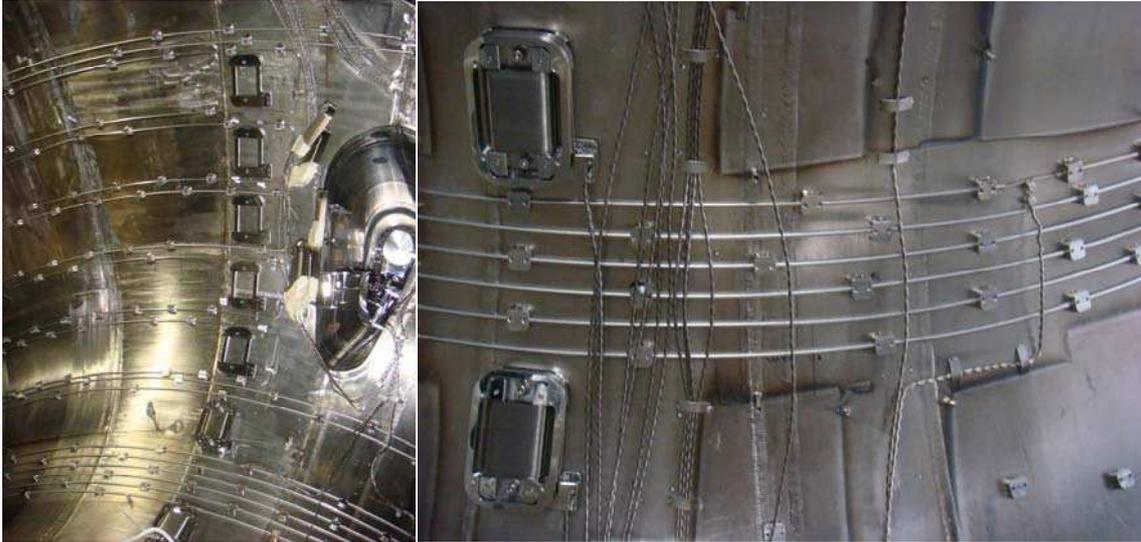
*Fig. 3. Installation of new magnetic diagnostics for 2009 and 2010 campaigns.*
